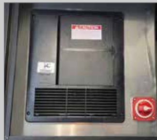
30 AMP COMBO LOAD CENTER WITH KILL SWITCH AND BATTERY INDICATOR
